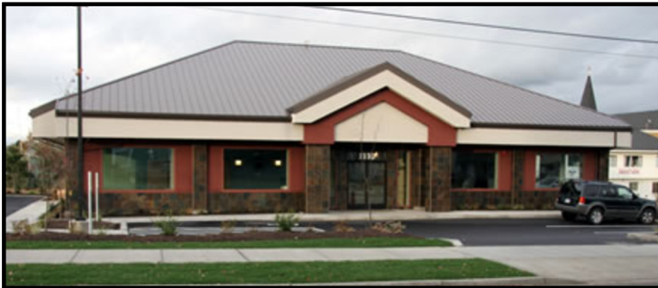
Renovation of the 22nd Street "Barto Building" Specialty Clinic
